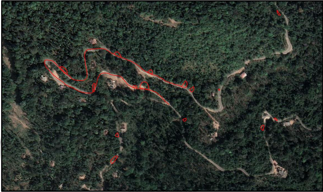
Fig. 7.2: Vulnerable zone at the hairpin bend on Bhagamandala-Talakaveri road
