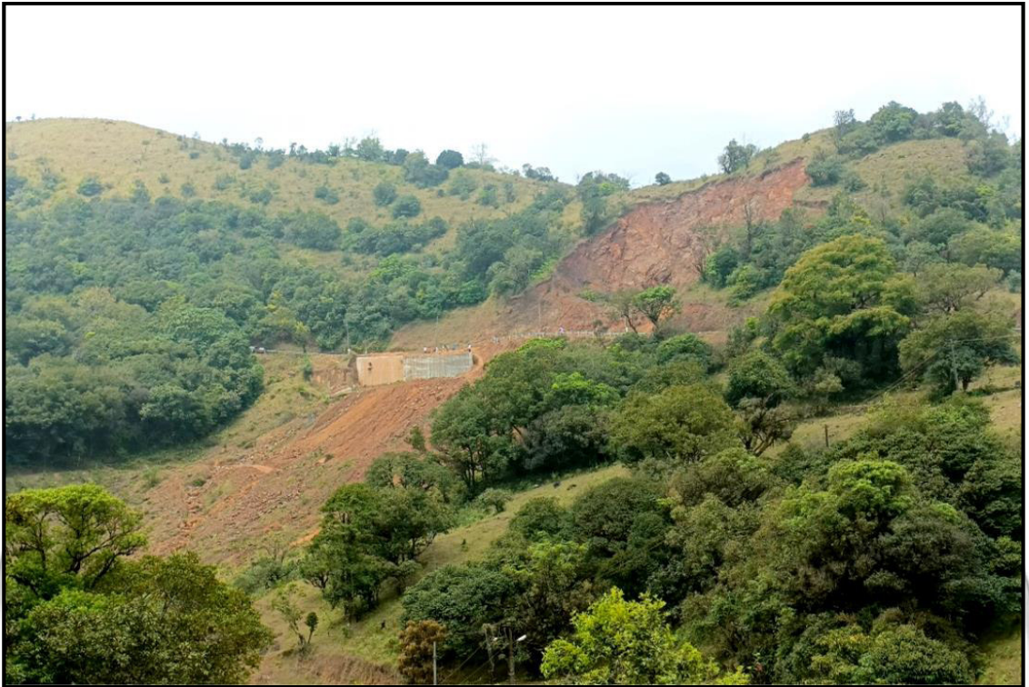
Fig. 4.1: A distant view of Talakaveri landslide
