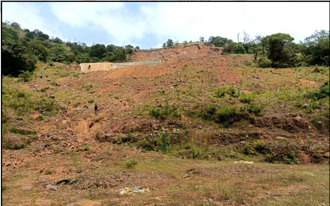
Fig. 6.6: Talakaveri landslide in the high susceptibility zone
