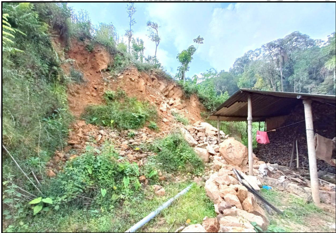
Fig. 4.4: Landslide initiated on a cut slope near a house in Cherengala
