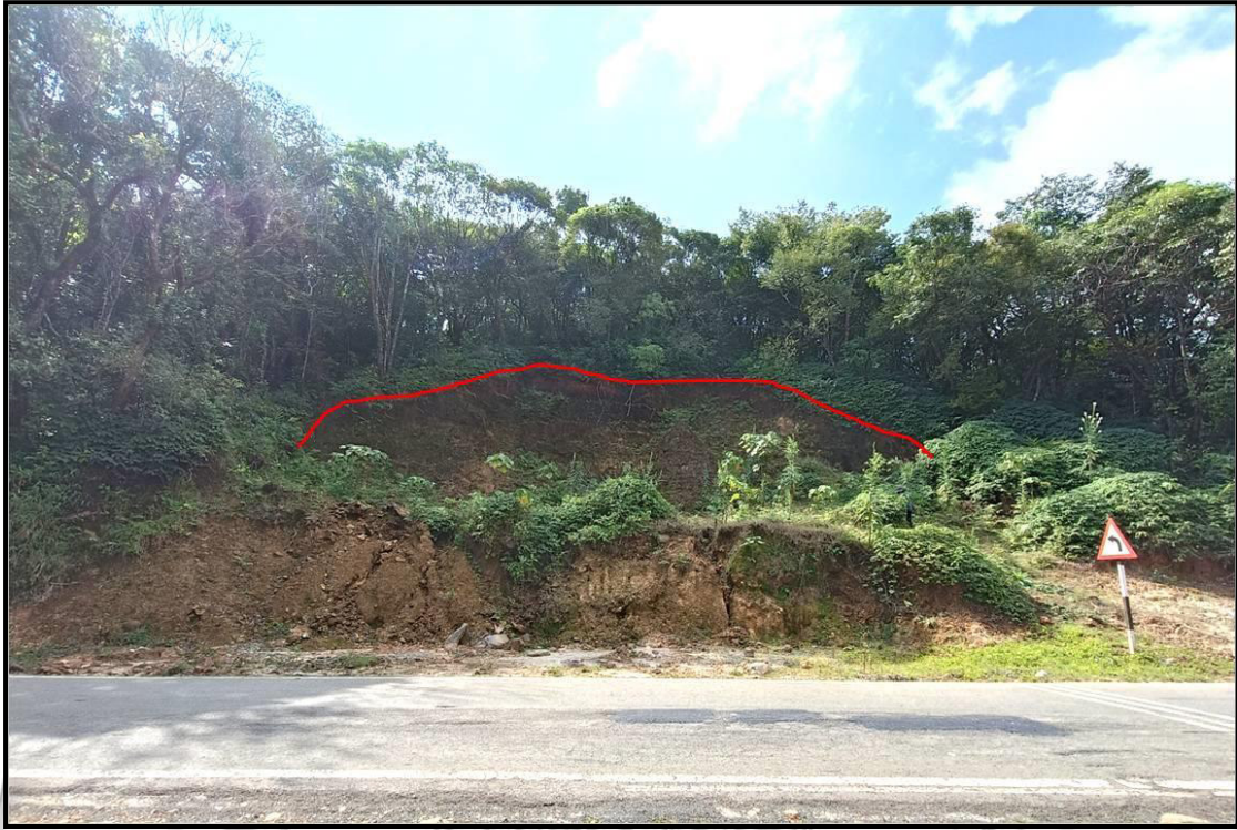
Fig. 4.3: A suspended landslide on Bhagamandla Talakaveri road
