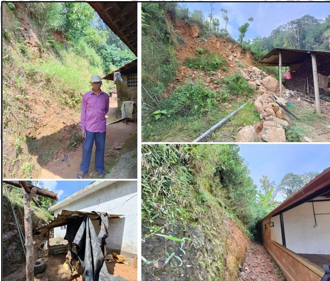
Fig. 7.4: Vulnerable houses near Cherengala
