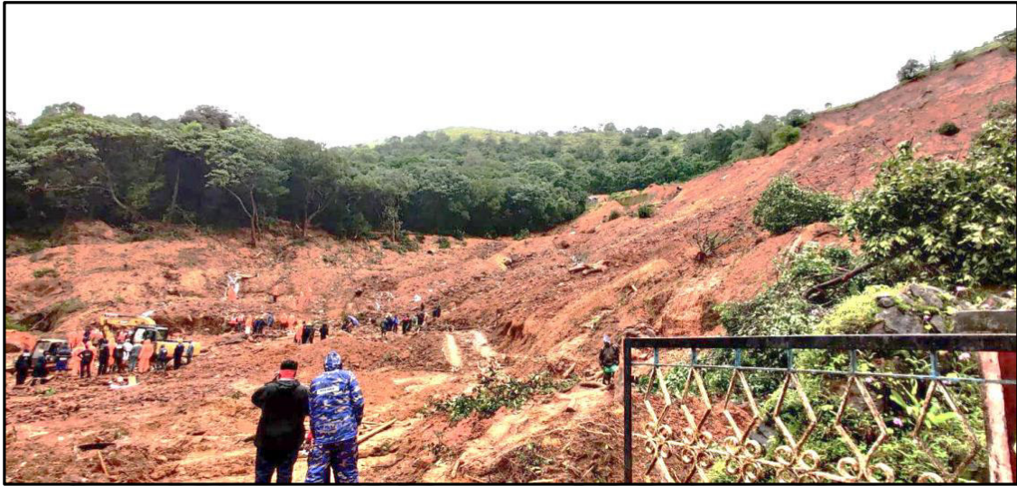
Fig. 4.8: A view of the landslide in 2020 (Source: 2020 GSI post-disaster report)
