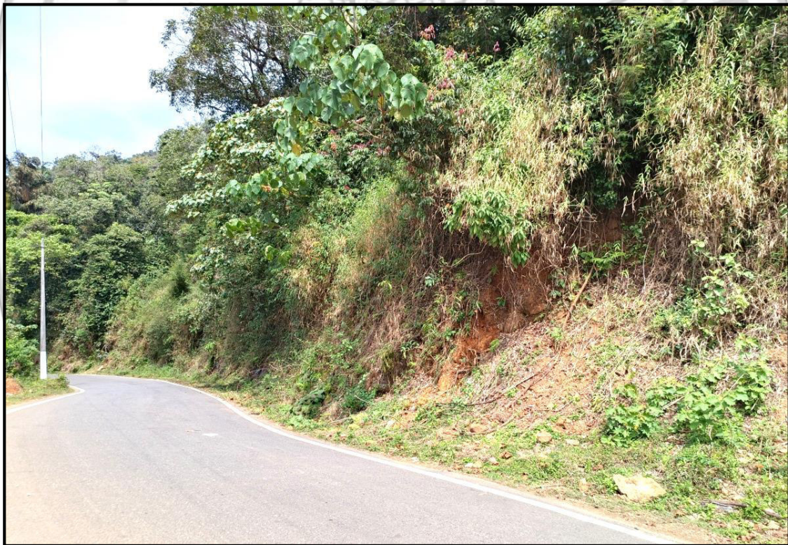
Fig. 6.7: A moderately susceptible cut slope on SH-90
