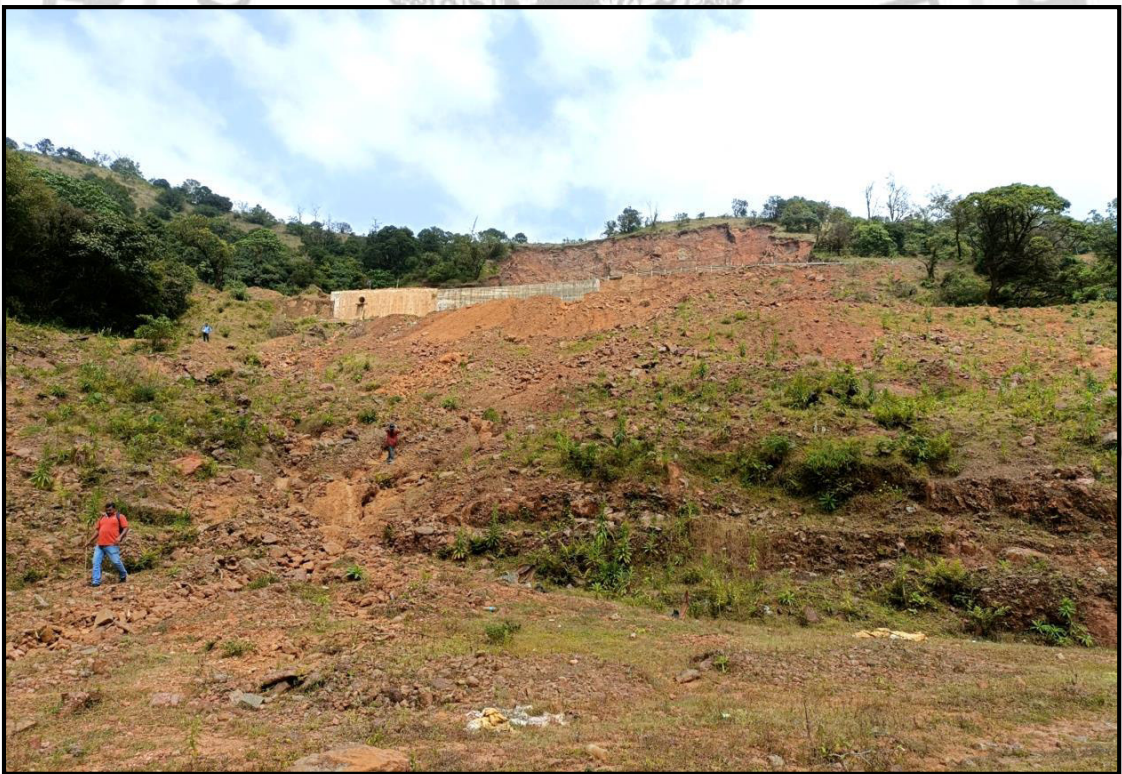
Fig. 5.19: Younger loose debris exposed in Talakaveri landslide runout zone
